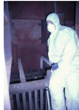
Above and Below: The flexi-lance is lowered into the area to be cleaned, and then the pressure wave is actuated
